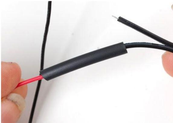
Shrink wrap tubing seals joint by heat from hair dryer.
